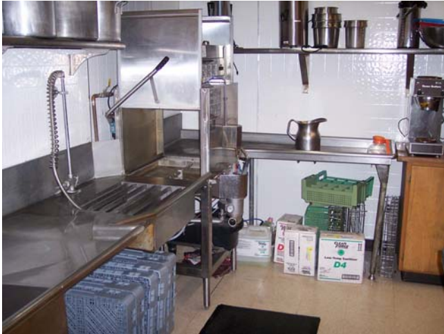
New walls, stainless steel sink & shelf, new floors
