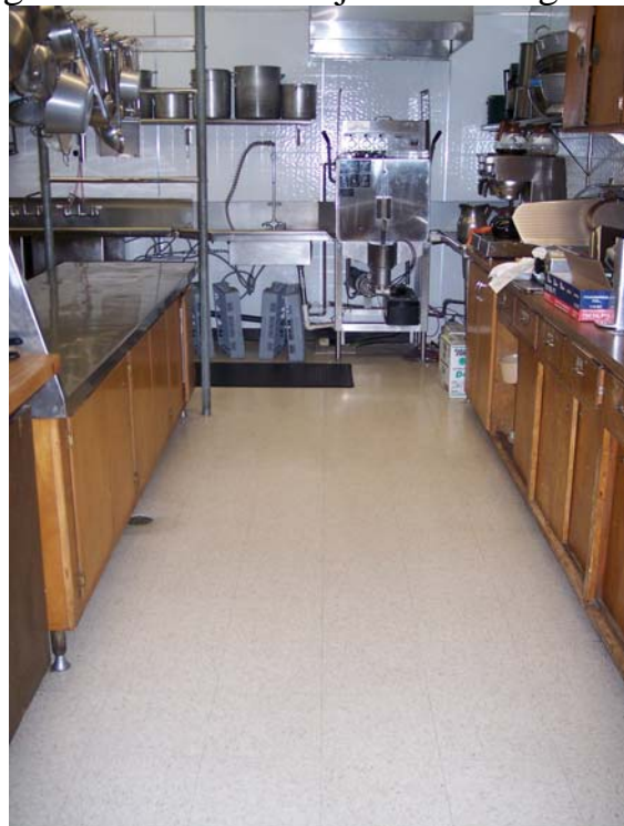
New kitchen floors, new walls and sinks
