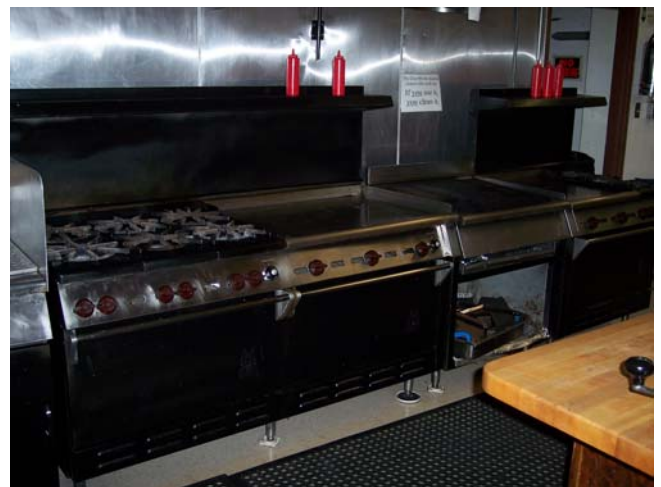
Refurbished kitchen equipment & butcher block
