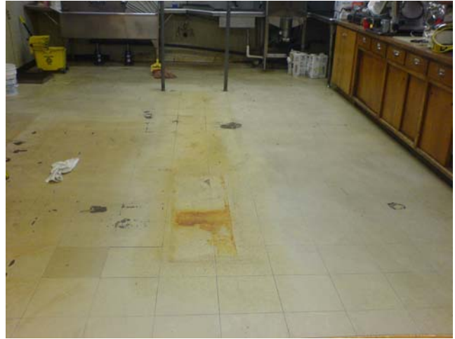
Old damaged kitchen floors also showing old sinks with car jacks holding them up
